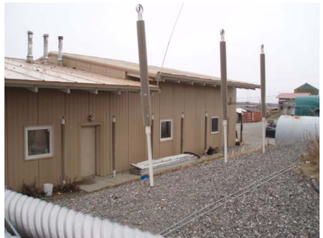
S04 WTP West Wall
