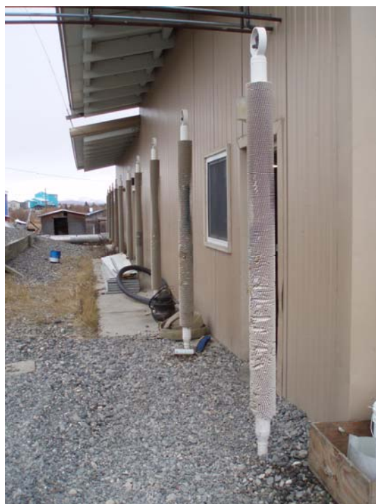
S06 Foundation Thermosiphons Along West Wall
