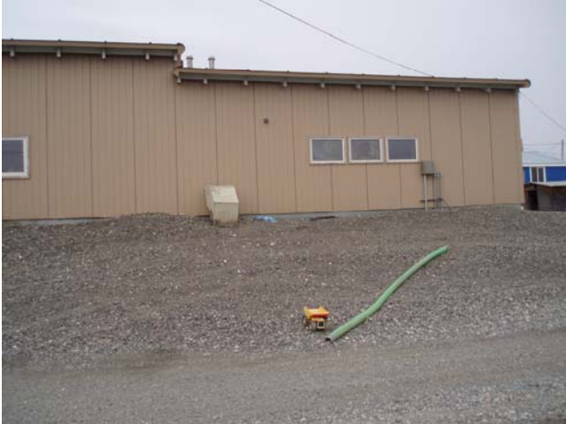
S03 Graveled Bank Along East Wall
