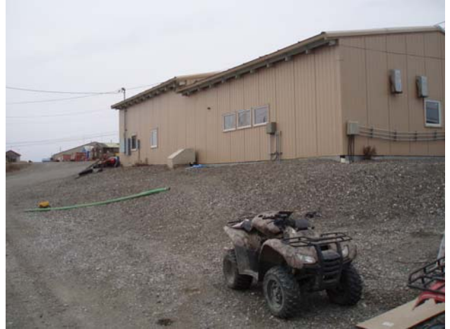
S02 WTP East Wall
