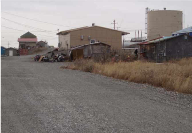
S01 Noatak WTP (Looking South)
