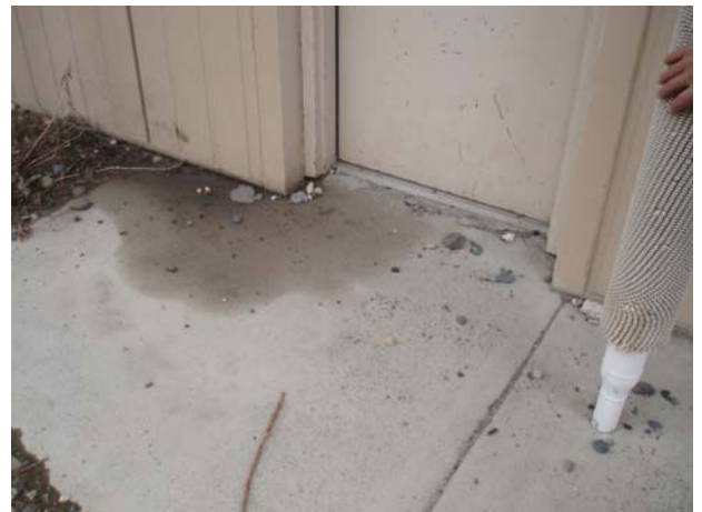
S16 WTP Entry Concrete Landing
