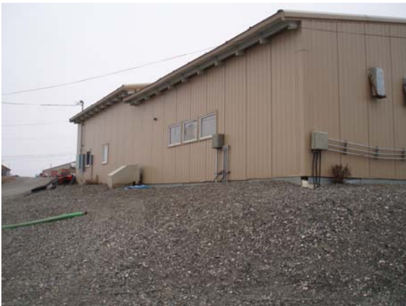
S15 Sloped Gravel Cover Over Water Circulation Lines to Community
