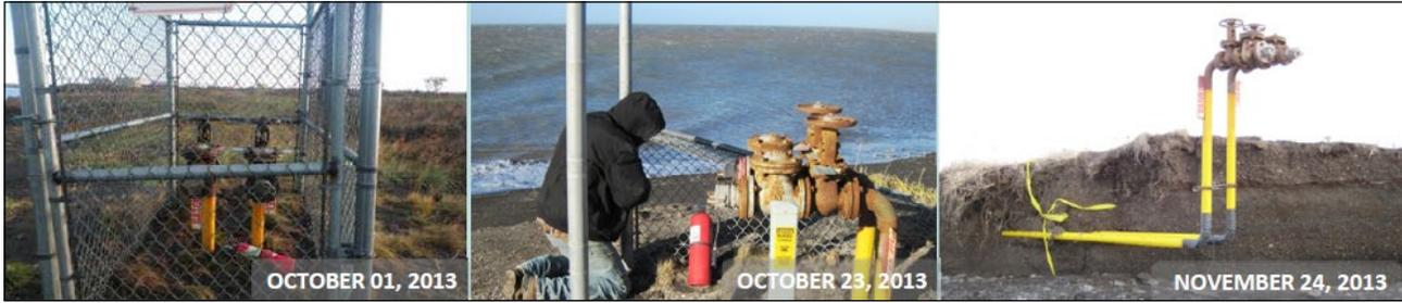
Figure 13. Fuel header pipes for Port Heiden's bulk fuel farm undercut by the eroding bluff during the 2013 storm season (photos by Linda Anderson, LEO).
