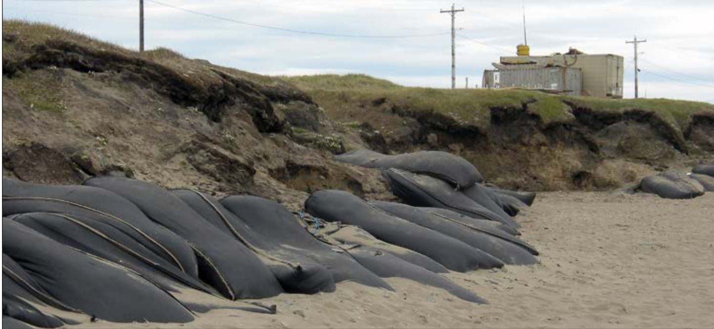
Collapsing bluff in Wainwright. Mike Brubaker, 2013.
