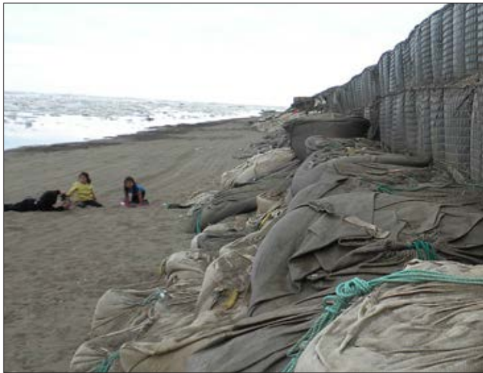
Wainwright revetment wall. Mike Brubaker, 2013.
