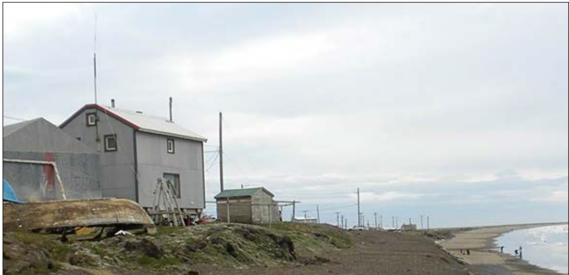
Beachfront: homes on bluff in Wainwright. Photo by Mike Brubaker, 2013.
