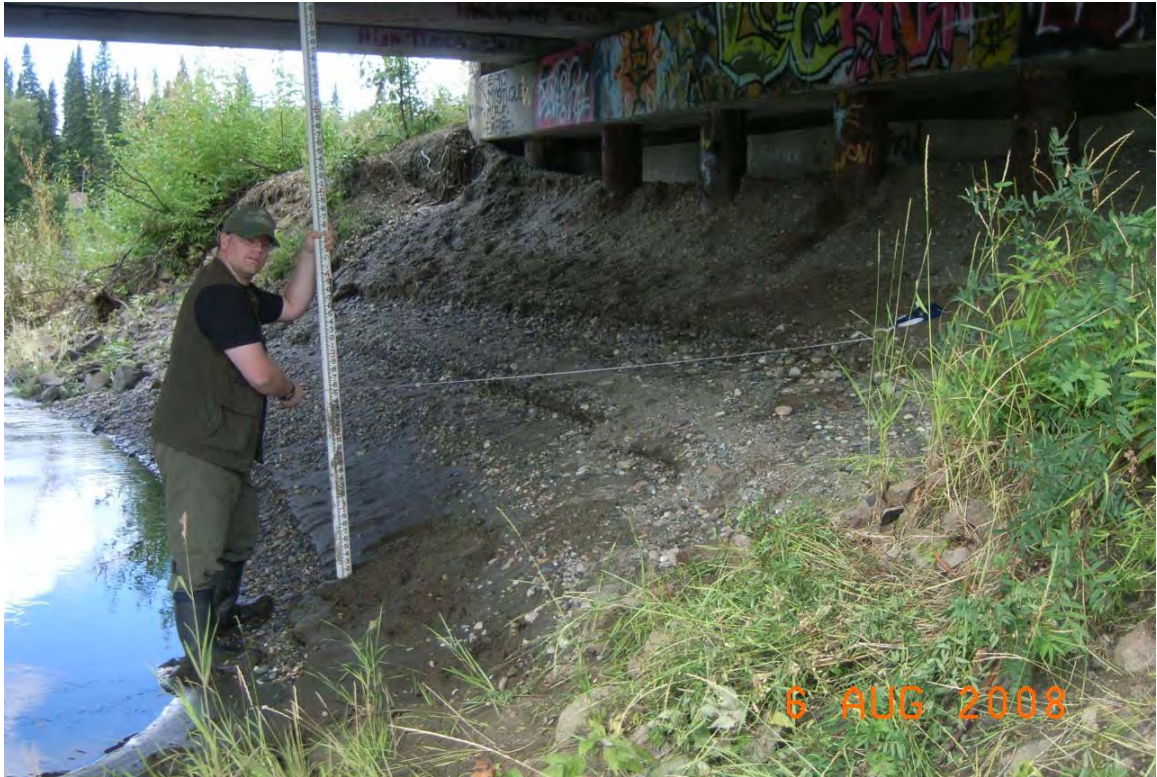
Figure 5: Erosion line on Chena River, Poor, North Pole, 2008.
