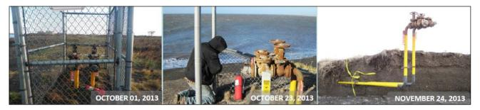
Figure 13. Fuel header pipes for Port Heiden's bulk fuel farm undercut by the eroding bluff during the 2013 storm season (photos by Linda Anderson, LEO).
