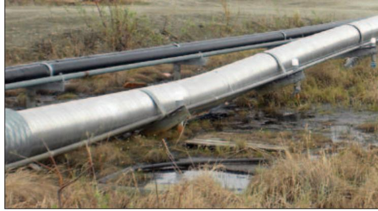
*Arctic pipes, sagging as they sink into the ground.
