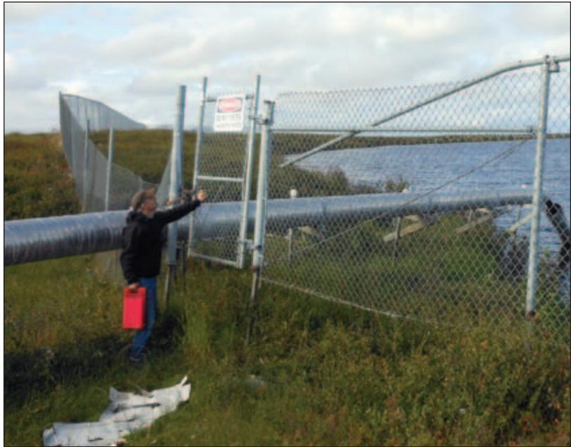
*Sinking and erosion has damaged the sewage pond outfall.
