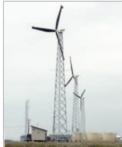
*AVEC's 65kw wind generators help power Selawik and control energy costs.
